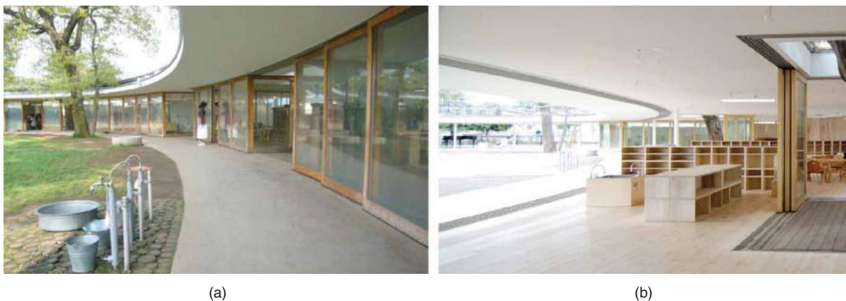
Figure 1. The classrooms of the Fuji Kindergarten designed by Takaharu Tezuka: (a) Classrooms are enclosed by patio doors but without walls, and (b) The patio doors can be fully opened to remove the boundaries of classrooms [9].
