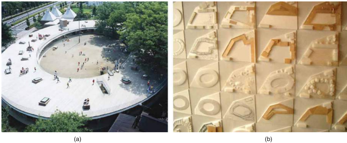
Figure 4. Geometric features of the roof of the Fuji Kindergarten designed by Takaharu Tezuka: (a) The geometric features of the roof consist of two simple ellipses, and (b) a series of mock-up models created by the architect [9].
