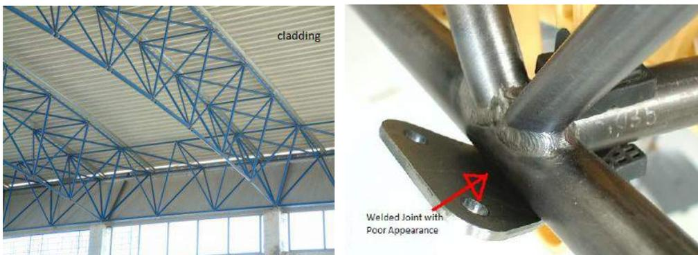
**Figure 3:** From left to right. (a) SF under Cladding, (b) Poor Appearance of Welded Joint in Conventional SF.
