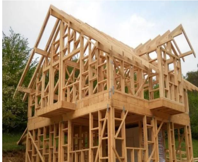
Figure 3: Assembled timber frame.
