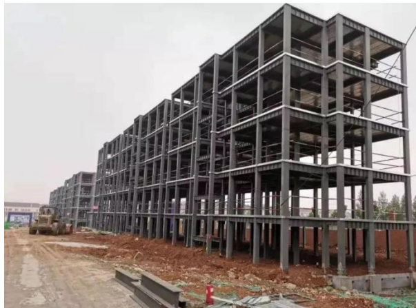
Figure 2: Assembled steel structure.
