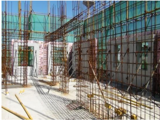
Figure 1: Assembled concrete structure.
