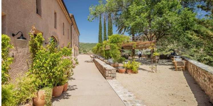
Figure 6: The scene after the reconstruction of the main entrance road of Tla Dominica Hotel (photo source: Muou Design network).
