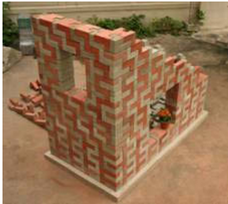
Fig. 12: Complete wall assembly made from blocks using cradle molding system.
