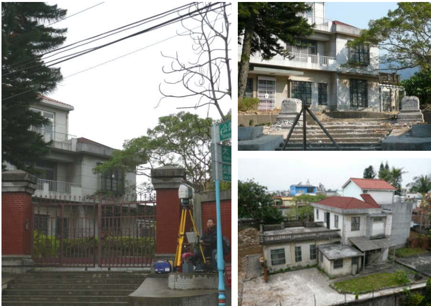
Fig. 1: The house before and in the middle of exterior renovation.
