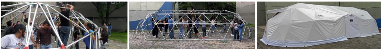
Figure 13. Assembly of the temporary structure with a rectangular base.
